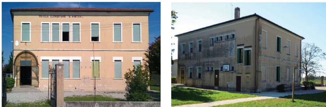
Figure 5. Front and back view of the A. Manzoni school.
