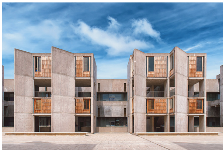
Fig. 3. Salk Institute for Biological Studies. Le cellule in teak conservate e ricollocate in opera ad intervento concluso (J. Paul Getty Trust 2017).
