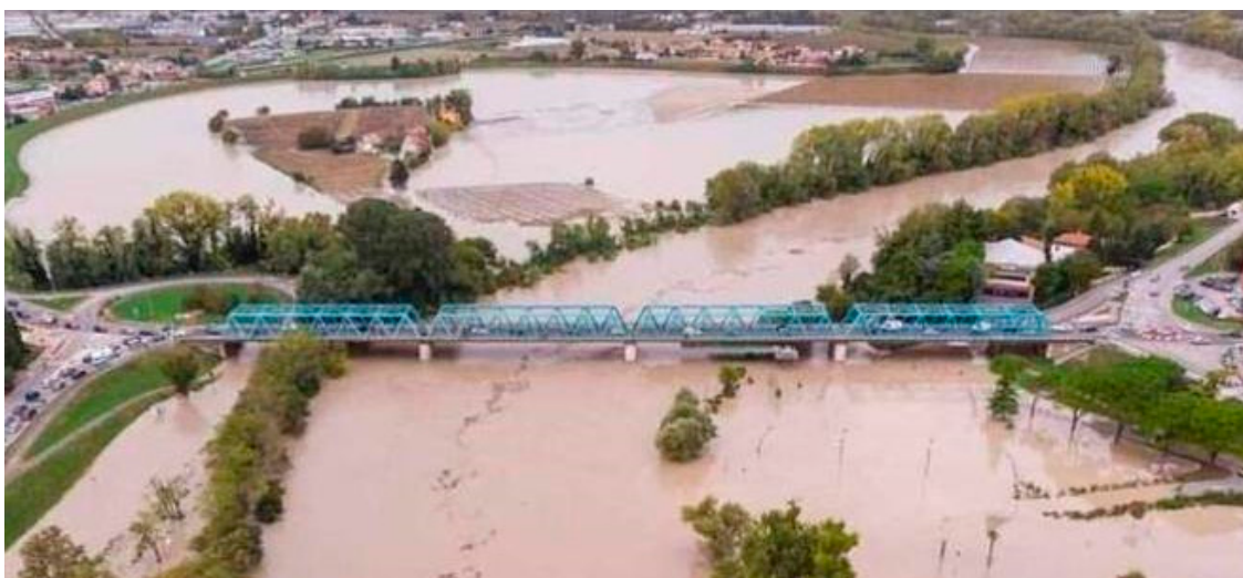
Figure 2. The November 2019 flood that flooded part of the territory of San Donà di Piave.
