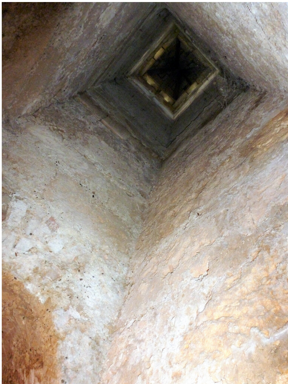
FIGURE 34 Irsina, Renaissance aqueduct called "Bottini". Detail of a spiraculo
