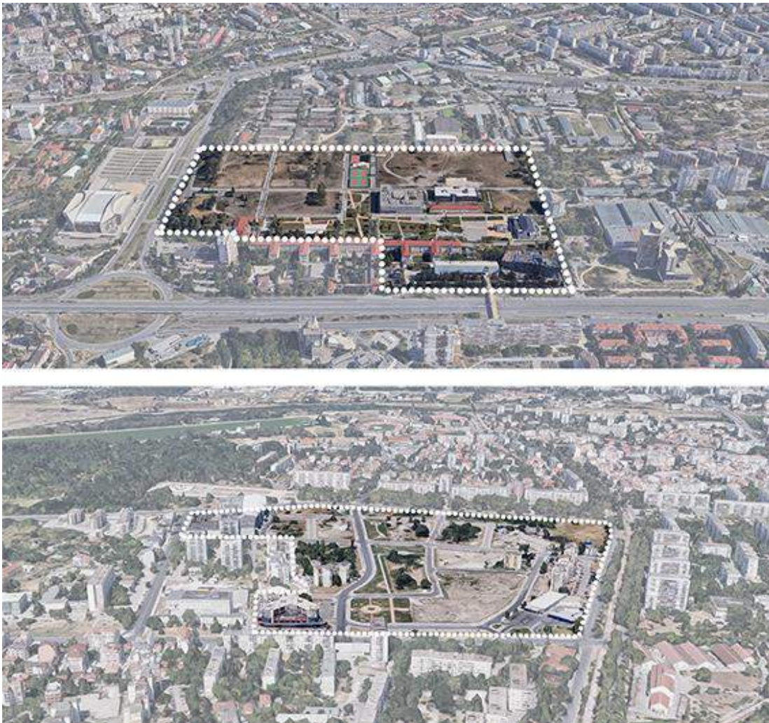
Figure 1: Aerial view of the case study areas in Sofia (above) and Plovdiv (below). Source of the base images: Google Maps, 2017.
