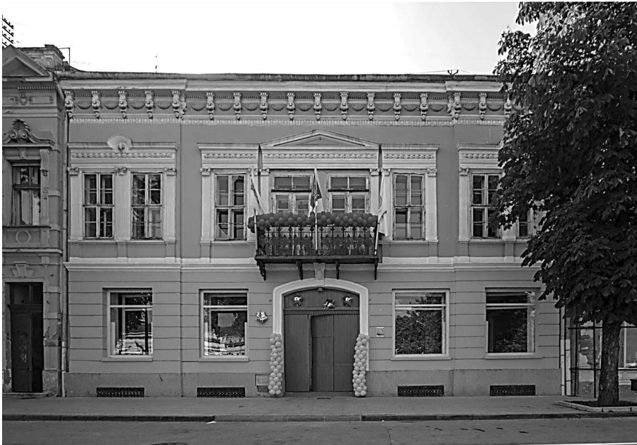
Figure 2. The front elevation of the revitalised Army Club. Source: photo by R. Peňa (2015)
