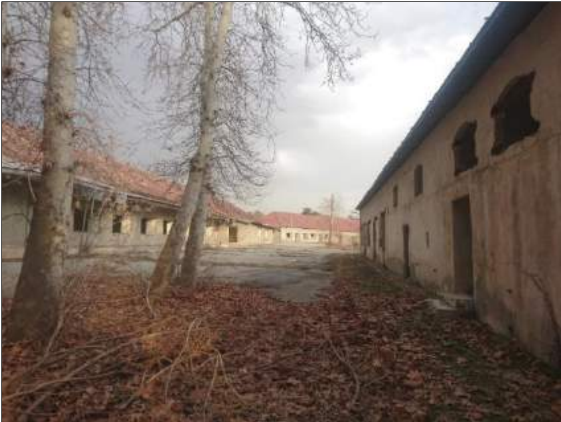
Figure 3. The Historical Buildings of O6 Barracks. Source: Authors
