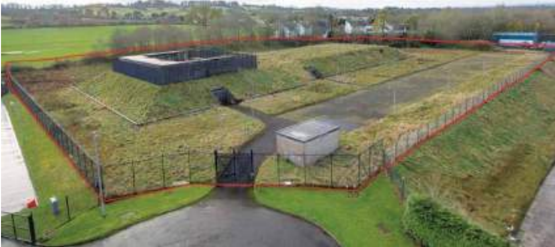
Figure 2. Ballymena RGHQ bunker as delineated in its sales brochure. Source: photo by Lambert Smith Hampton (2016)
