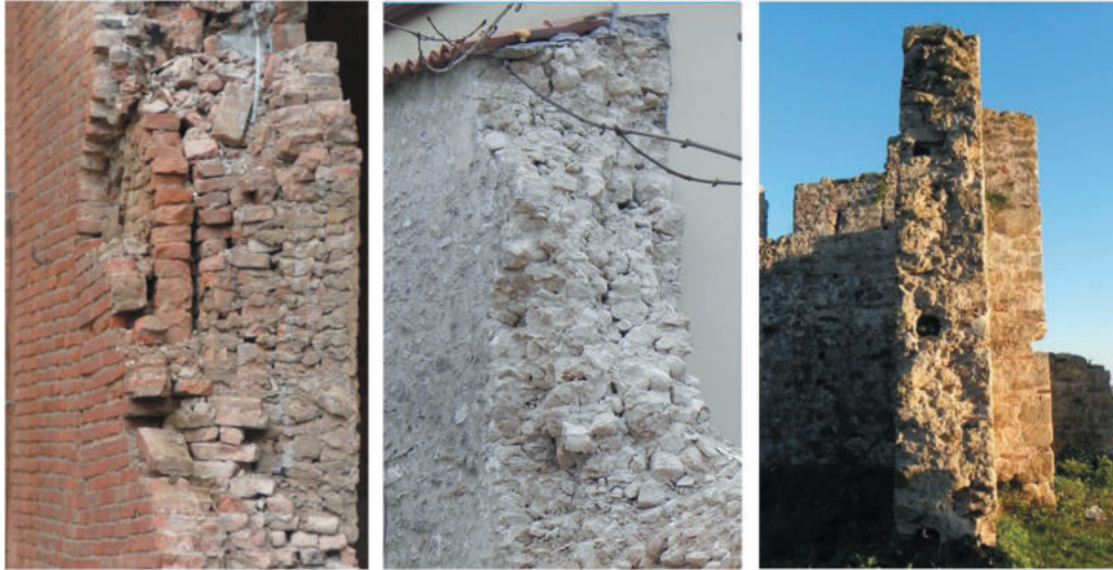
Figure 3. Instantiating cross sections of walls. From the left: Rocca di San Felice sul Panaro (Emilia); Norcia curtain wall (Central Italy); Bashtove Castle (Albania).
