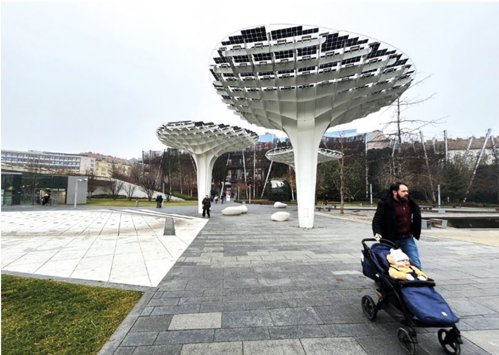
Fig.02 The solar canopy structures at Millenàris Park offer shade, cooling, and renewable energy, while the open, accessible pathways support inclusive, family-friendly urban design.
