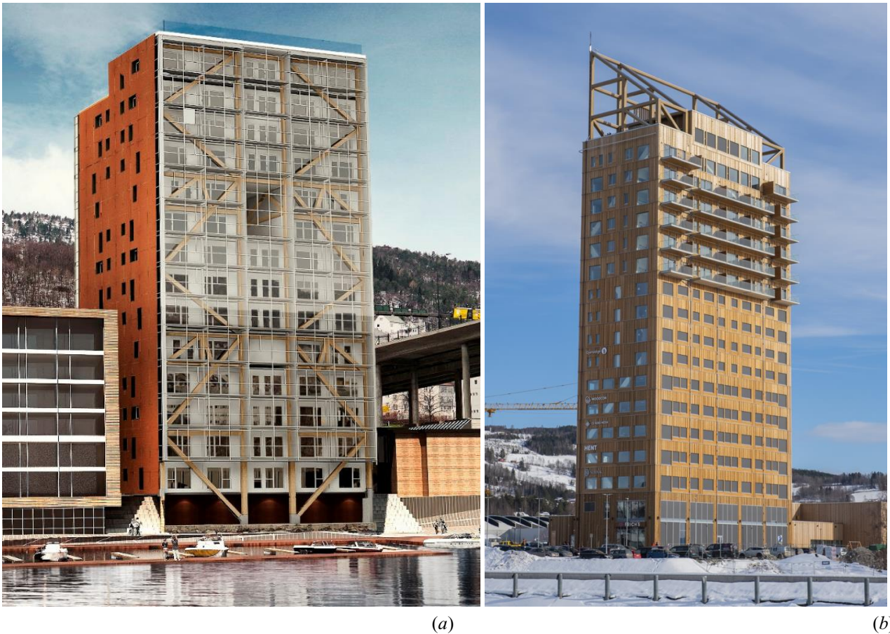
Figure I.1-2 – High timber buildings in Norway: (a) Treet and (b) Mjøstårnet ( image credits: (a) Abrahamsen & Malo [18] and (b) Moelven website [30] ).
