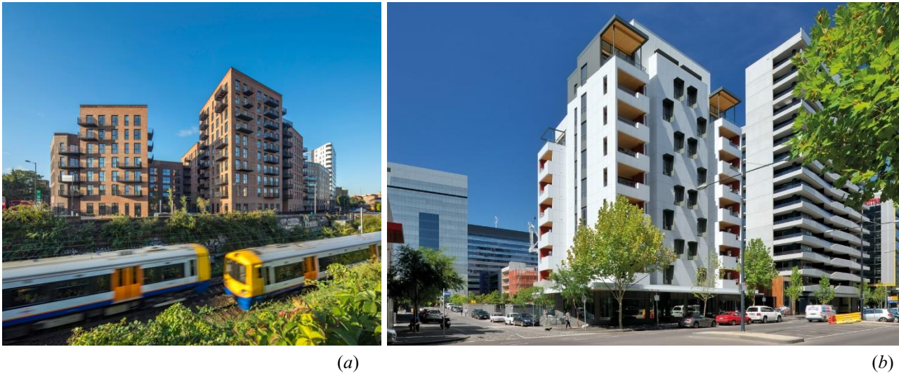
Figure I.1-1 – CLT multi-storey timber buildings: (a) Dalston Lane building in London (United Kingdom) and (b) Forte building in Melbourne (Australia) ( image credits: (a) Waugh Thistleton Architects website [15] and (b) The Possible website [16] ).
