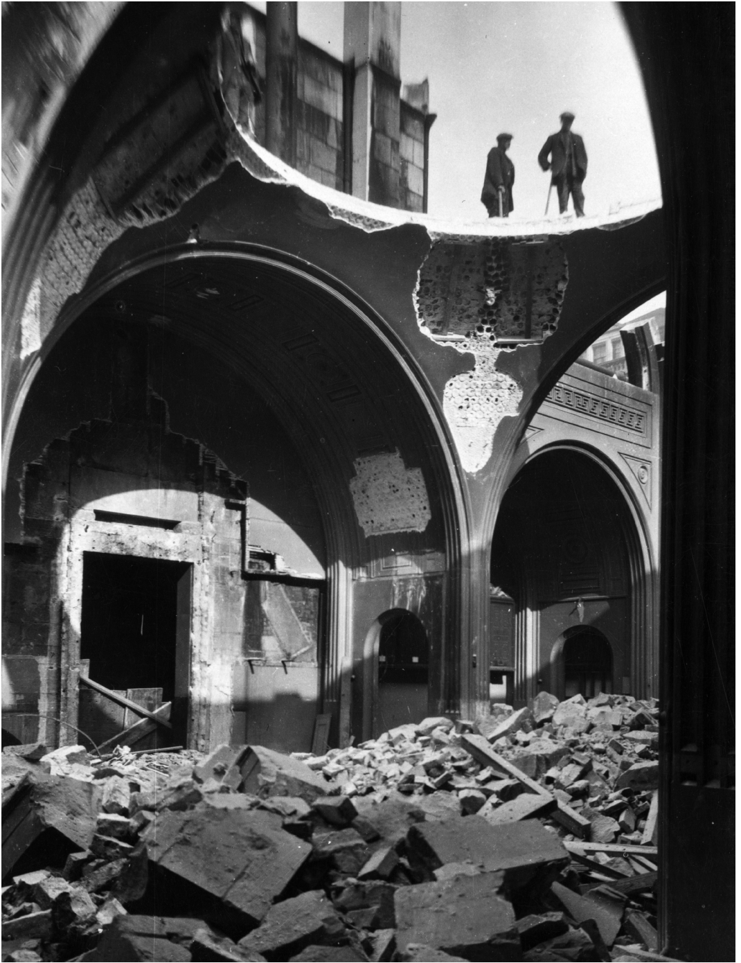
The Bank of England, Threadneedle Street, City of London: the Old Dividend Office during demolition
