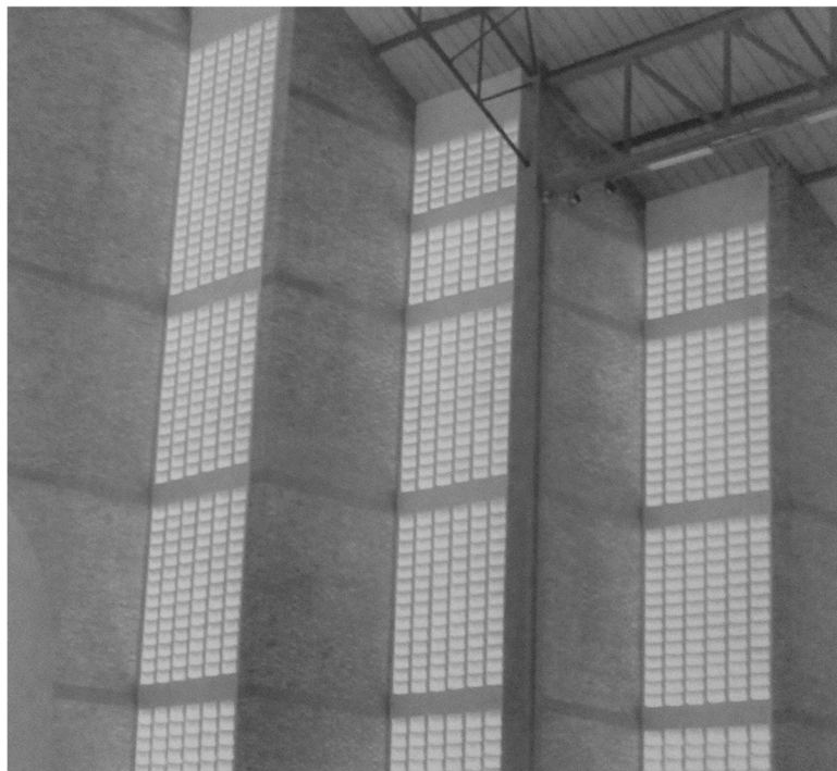
FIGURE 146: DETAILS AND EXECUTION OF THE CLAUSTRAS IN BUJUMBURA (SACRE-COEUR CHURCH), SOURCE: ARCHIVES OF PAUL DEQUEKER, KADOC
