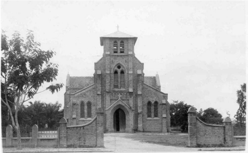
FIGURE 83: SAINT ANNE'S CATHEDRAL BUILT AROUND 1930 IN LEOPOLDVILLE, SOURCE:
