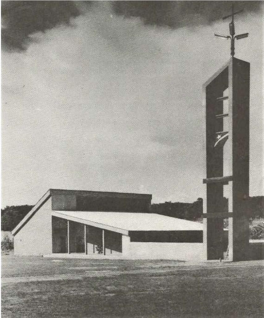
FIGURE 94 ; CHAPEL OF THE NGANDA CENTER IN KINSHASA, AN EXAMPLE OF MODERNISM APPLIED BY PAUL DEQUEKER: PHOTO: PAUL DEQUEKER, SOURCE KADOC
