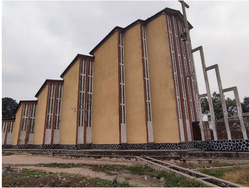
FIGURE 223: CONTRARY TO THE ORIGINAL IDEA OF THE ARCHITECT PAUL DEQUEKER, WHO USED UNPAINTED WALLS, THE WALLS ARE NOW PAINTED. PHOTO: VICTOR BAY 2021
