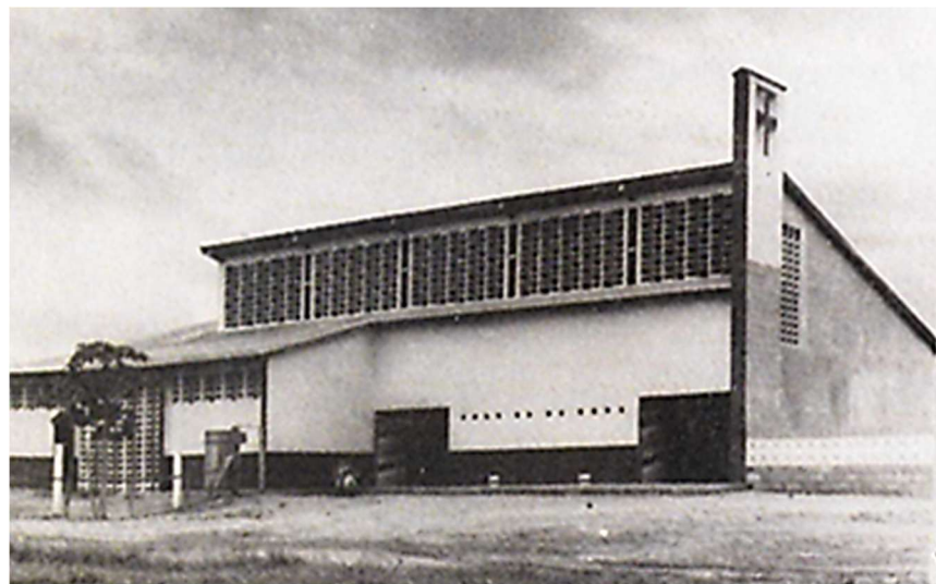
FIGURE 136: SAINT MATHIAS OF BUMBA, 1964, SOURCE: ARCHITECTURE TROPICALE
