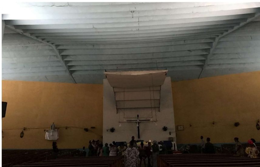
FIGURE 167: THE LOOK OF THE LONG-SPAN TRUSS THAT ALSO SERVES AS A CEILING, PHOTO: VICTOR BAY 2021
