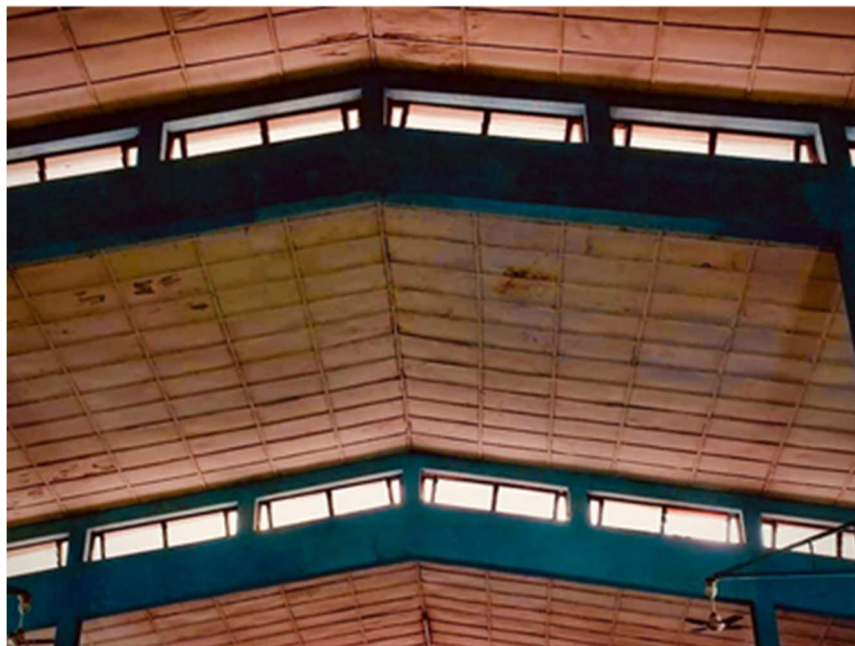
FIGURE 221: TOP VENTILATION TRANSOM WINDOWS ALSO ALLOWING NATURAL LIGHTING, PHOTO BY VICTOR BAY, 2021
