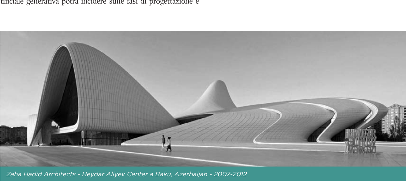
Zaha Hadid Architects - Heydar Aliyev Center a Baku, Azerbaijan - 2007-2012
