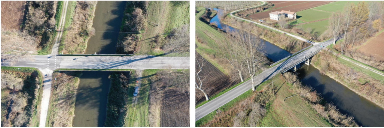
Figure 1. Fratta bridge (Italy): aerial views obtained with the drone survey.
