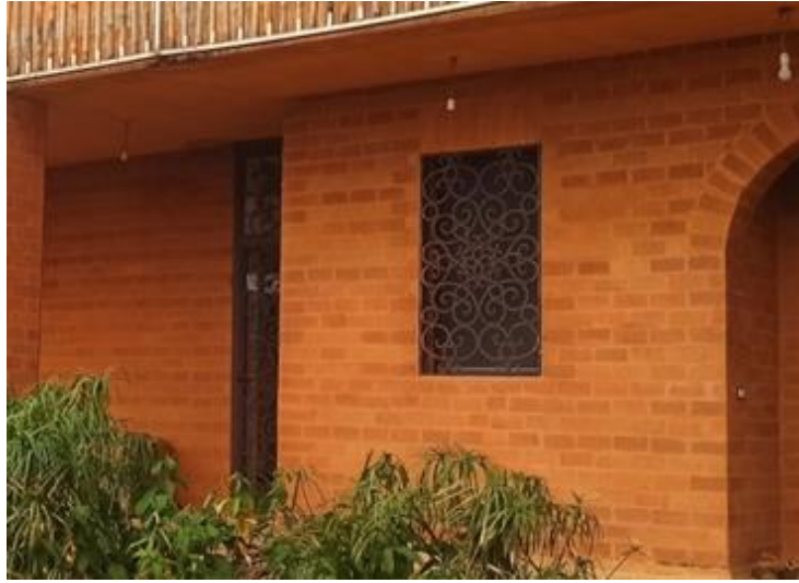
Figure 2.8: Earth-based mortar in earthen masonry house, Senegal.
