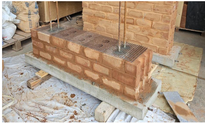
Figure 4.6: Positioning of the BFRP reinforcement net within the bed mortar joint.
