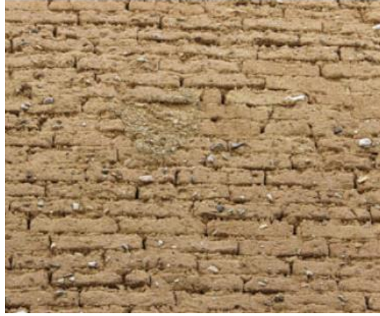
Figure 2.6: Adobe masonry wall with coarse aggregates, from [9].
