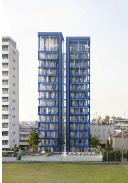
Figure 89 Note the two blocks separated by the usual transparent core, a response to building regulations, as well as the difference in scale of the attic and the privacy ensured by the clear separation of the units. Demogo's Xlam tower (2019).
