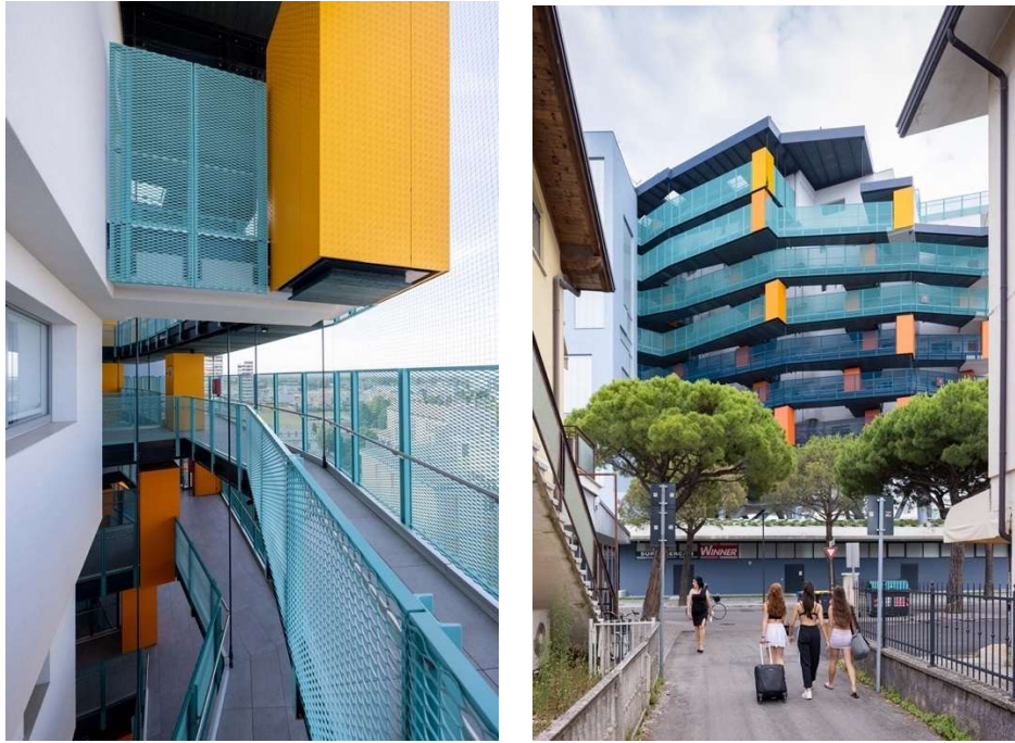
Figure 102 Podium exterior access balconies and elevator (2021).
