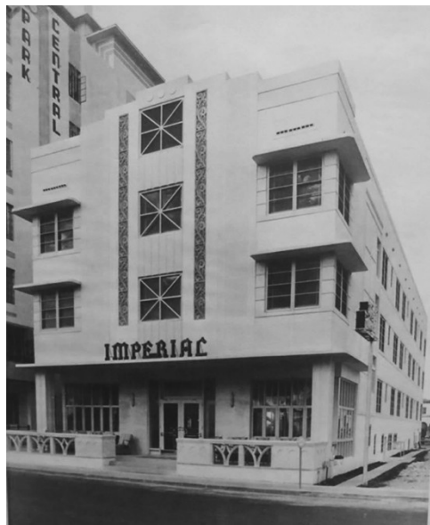
Figure 22 The Imperial Hotel in Miami clearly reveals the prominence of the front porch and its relationship with the adjoining street, as well as the contrast between the façade and the rear building mass.(c.1930).
