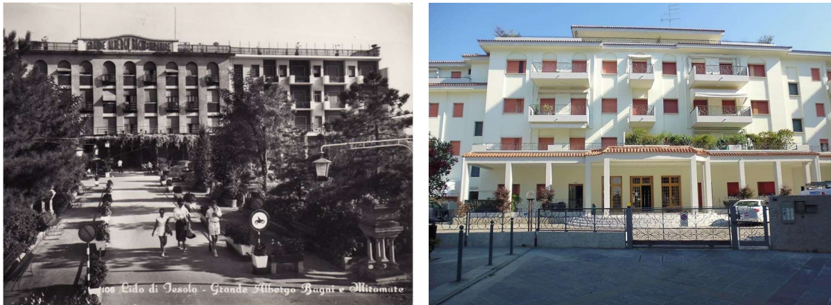
Figure 60 Grand Hotel Bagni & Miramare before (c.1950) and after (today) its transformation into a residence.
