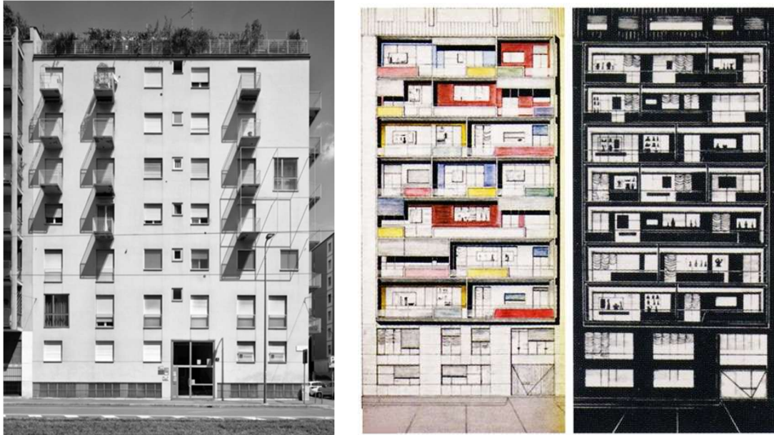
Figure 18 On the left: a photograph of Asnago Vender's condominium on Via Faruffini (1953–54) by Marco Invernizzi. On the right: drawings of Gio Ponti's buildings on Via Dezza (1956–57), illustrating the flexibility of the facade framework and the importance of transparency as a compositional element, particularly in the building's nighttime appearance.
