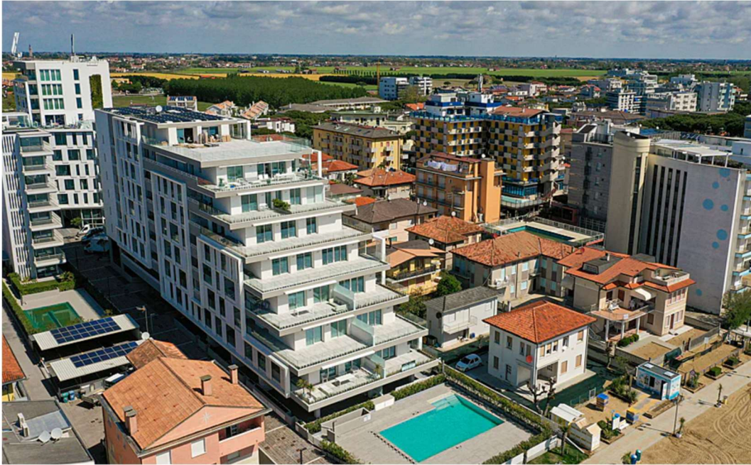
Figure 70 Tahiti after completion (2023).
