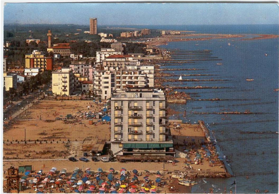
Figure 56 Postcard of Jesolo Lido showing the 1966 flood that completely washed away the beach. In the background, the recently constructed Pineta Tower is visible (1966).
