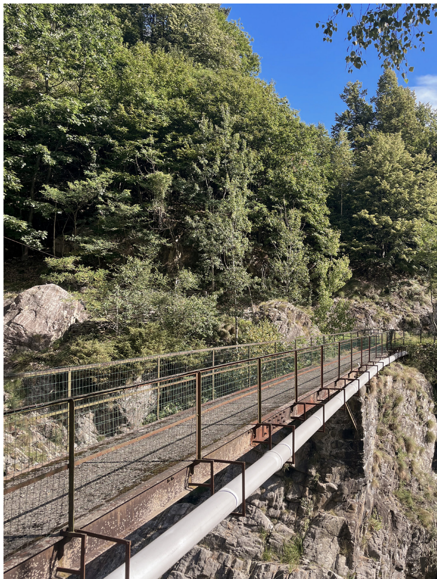
fig.10.28 Small infrastructures originally serving the mining sites have been converted for maintenance purposes and to provide access along the hiking routes. Isola di Vocca ( photograph by the author, 2023 ).
