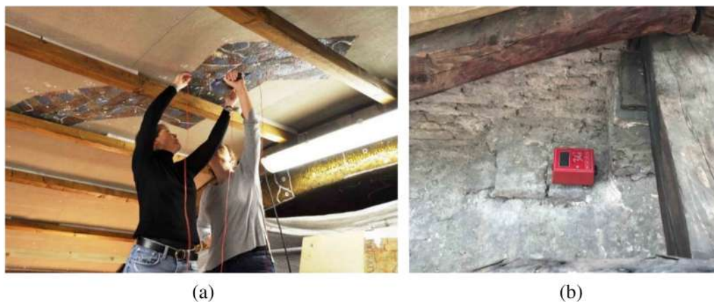
FIGURE 5 In situ measurements using (a) sonic testing and (b) tromograph device
