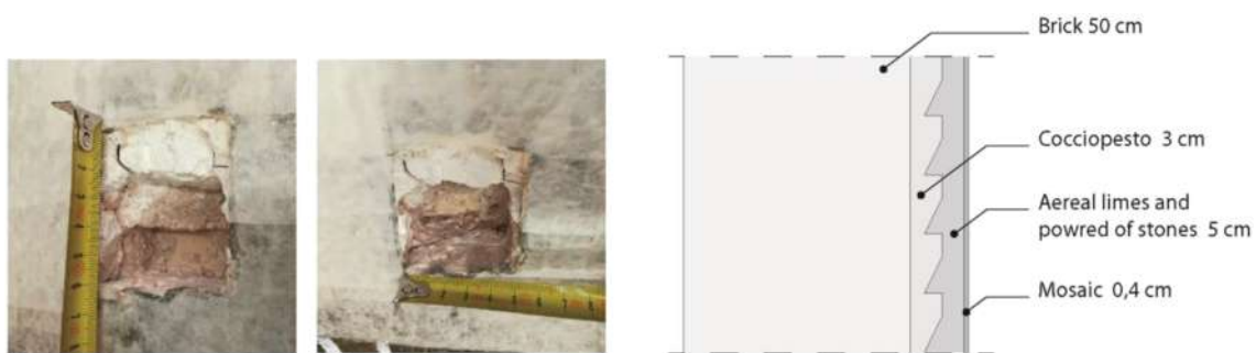
FIGURE 3 Masonry stratigraphy
