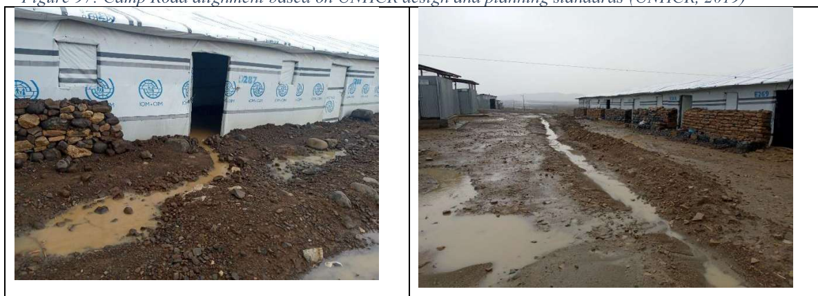
Figure 98: Poor drainage conditions in SC4 Mekelle during rainy season 2023 (Source: author 2023)
