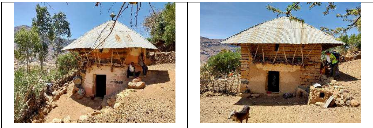
Figure 175: Variations of hidmo housing with adapted roof materials in Bora, South Tigray (Source: author, 2024)
