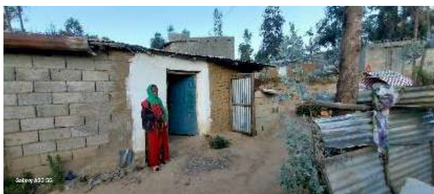
Figure 146: Mud block shelter constructed by an IDP on a host family's plot in Adigrat (Source: author, 2024)
