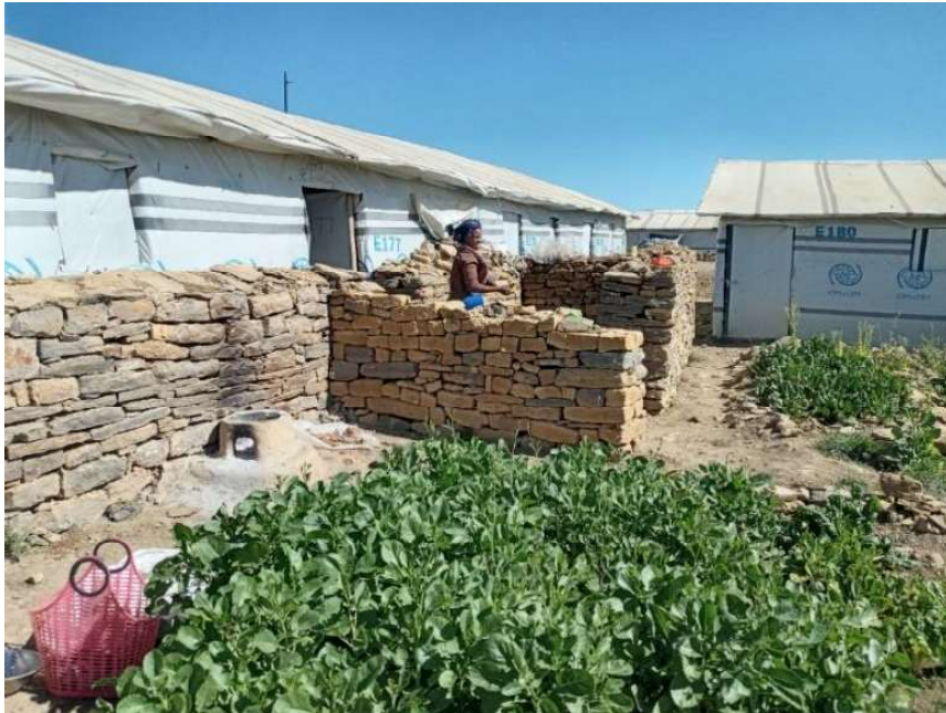
Figure 104: Transformation and adaptation of shelter and additional space using traditional dry-stone masonry (Source: author, 2023)
