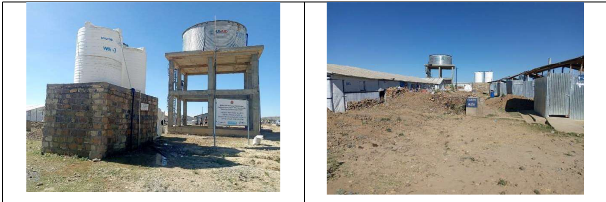
Figure 91: Elevated water reservoir (Source: author 2023)
