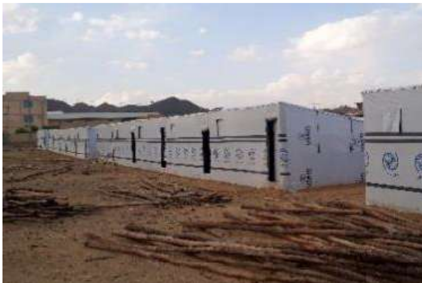
Figure 47: Modular shelter units in Shire area (Source: ESNFI Cluster, 2022)
