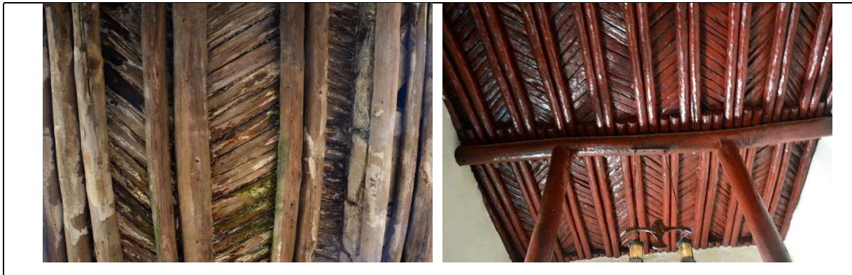
Figure 170: Typical Hidmo ceiling in Aynalem, Mekelle (Source: Patassini D., 2023)
