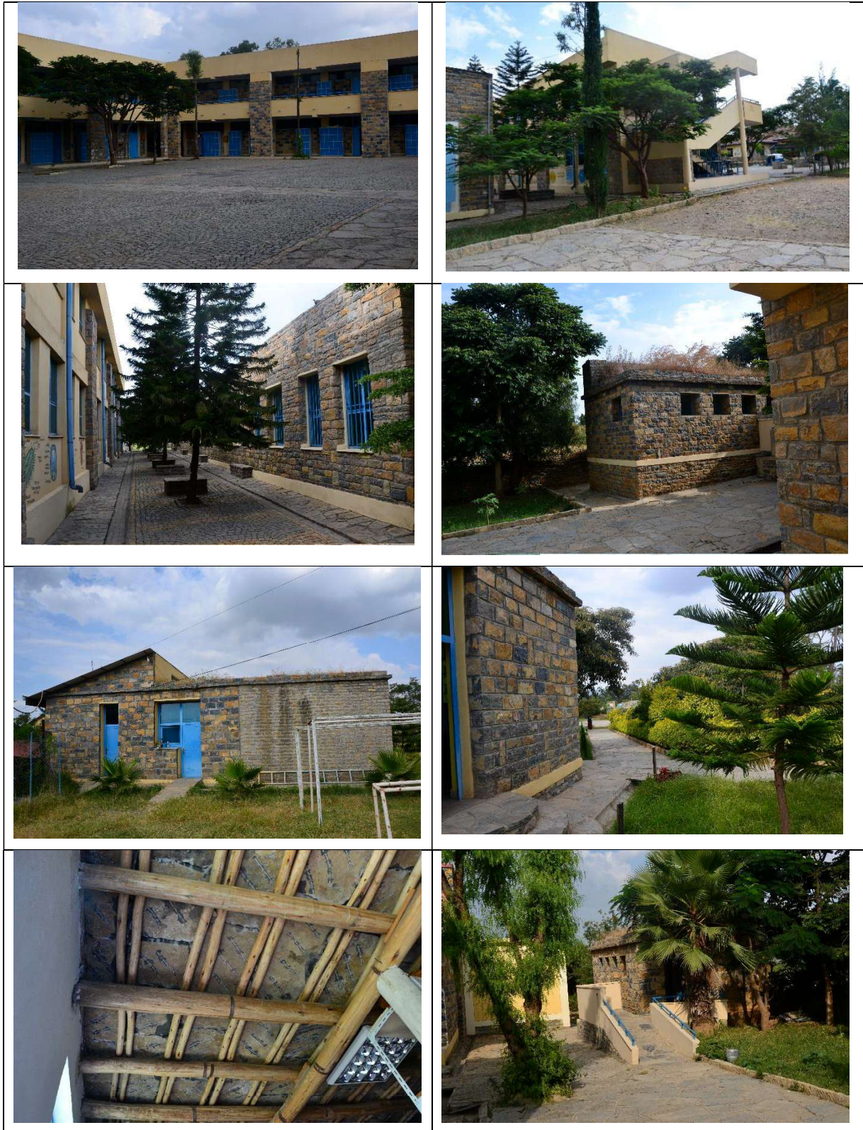
Figure 192: Integration of modern design with traditional hidmo technology at Nicolas Robinson School in Mekelle (Source: Patassini D., 2025)
