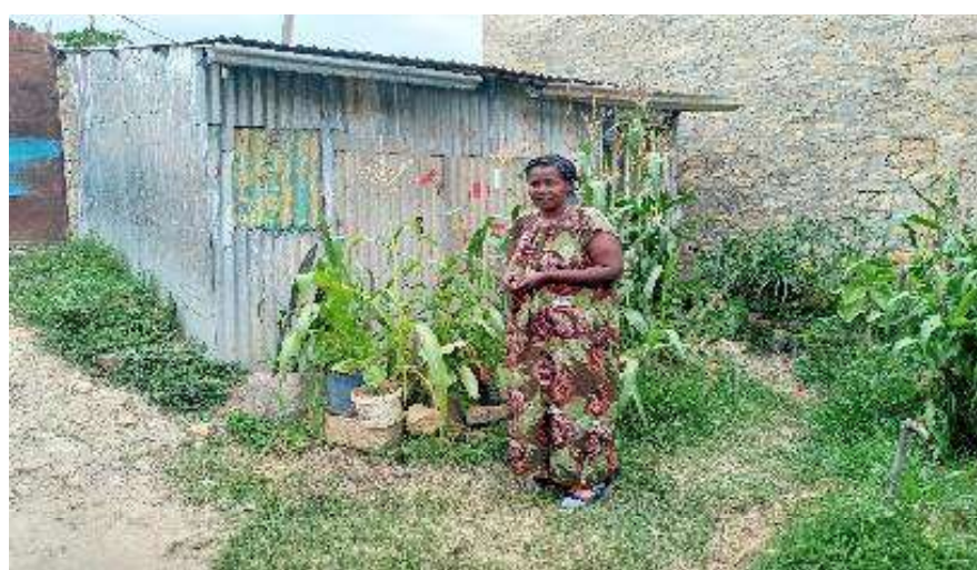
Figure 147: CGI shelter constructed by an IDP household on a host family's plot in Mekelle (Source: author, 2022)
