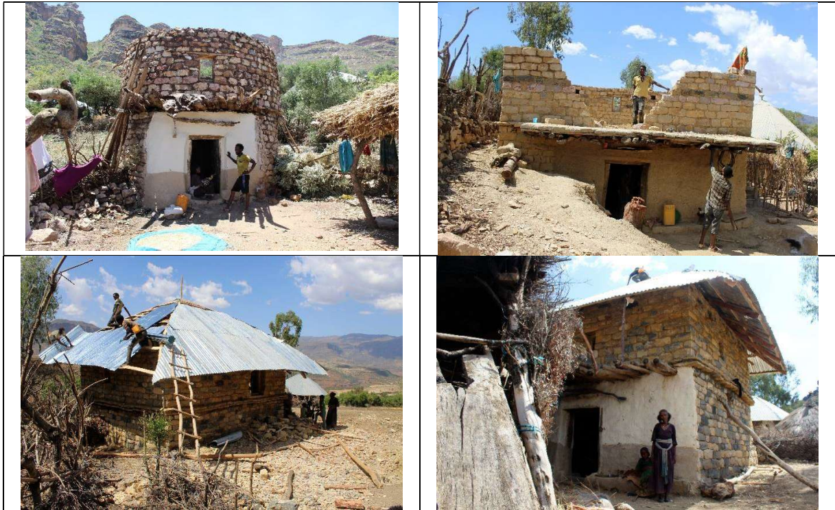
Figure 165: Reconstruction of damaged house in Bora area, South Tigray (Source: author,2024)
