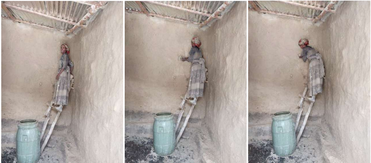
Figure 166: Wall plastering: women’s participation in post-war housing reconstruction in Bora town, South Tigray (Source: author,2024)
