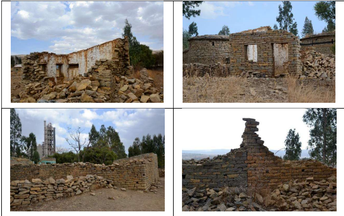
Figure 188: Demolished Hidmo house on the outskirts following industrial developments in the Messebo area of Mekelle (Source: Patassini D., 2024)
