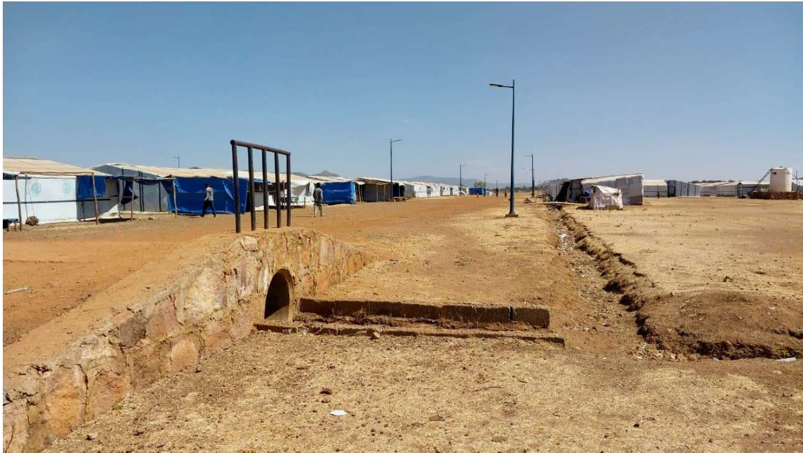
Figure 123: Site improvement in the camp (Source: author December, 2025)
