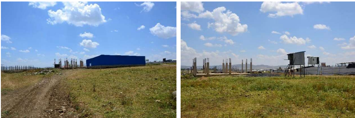
Figure 110: Industrial building/garage under construction adjacent to the camp (Source: Patassini D. 2025)
