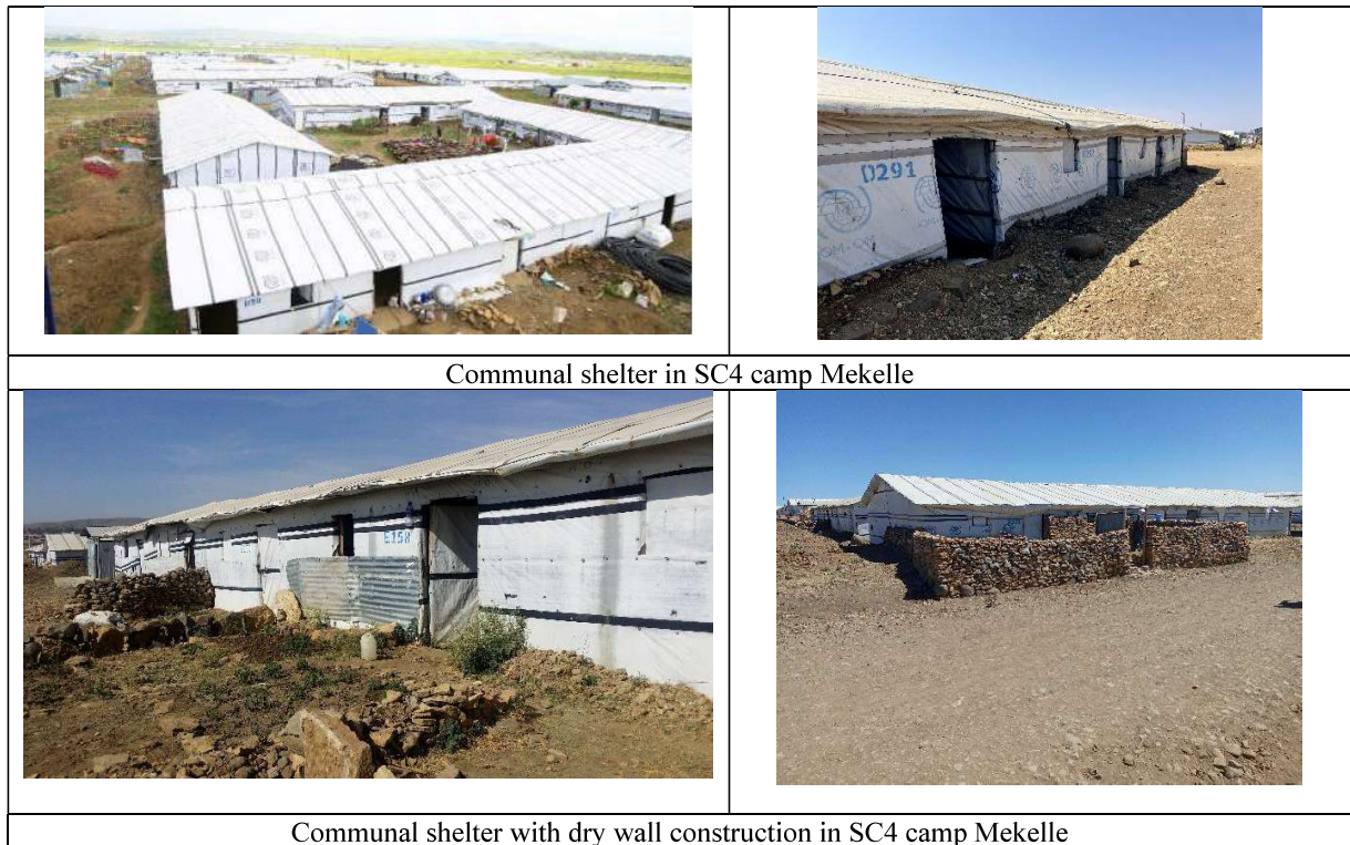
Communal shelter with dry wall construction in SC4 camp Mekelle
