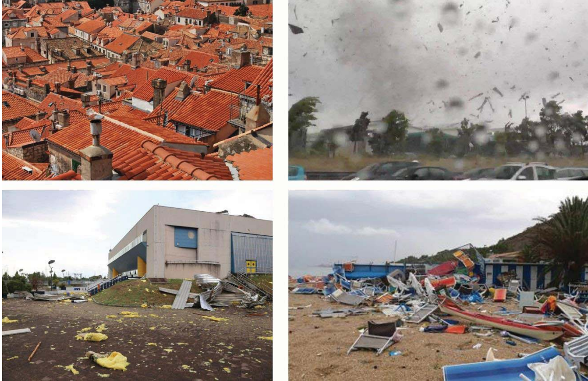
Figure 3. The context assessment is essential to identify the possible risks and the elements that can fail in case of strong winds, becoming flying debris.
