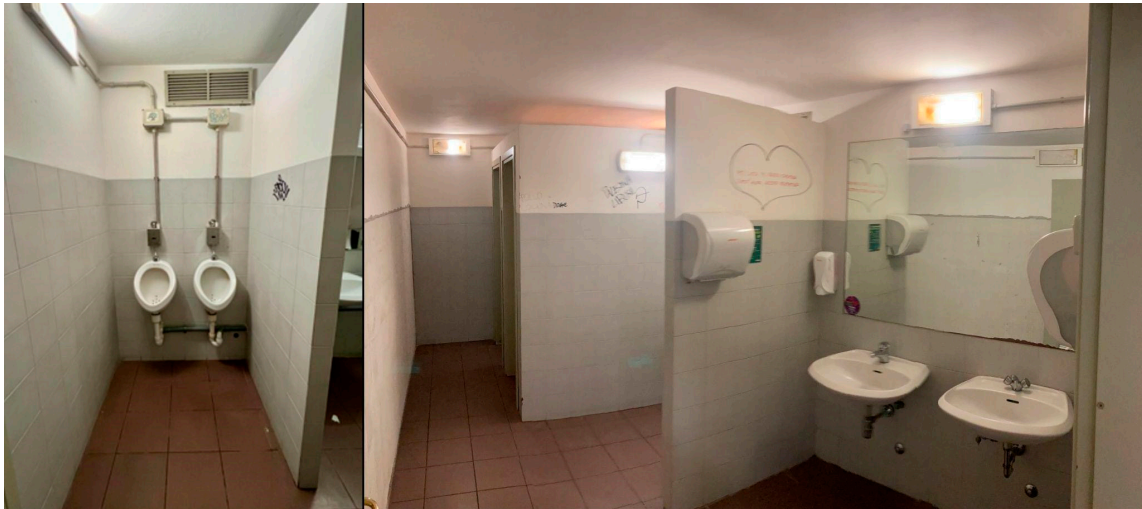
Figure 3. (left) The urinals available in the un-renovated restrooms are too close to each other, making their simultaneous use unpleasant from a privacy point of view and almost impossible from a physical point of view. (right) Un-renovated male restroom image from the entrance.
