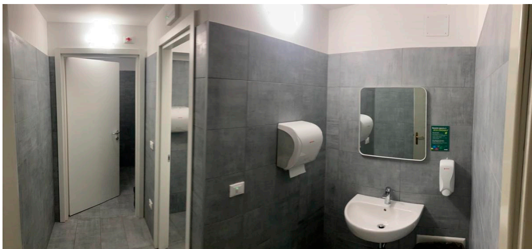
Figure 4. Renovated toilets on the ground floor. They present two cubicles and only one washbasin in the vestibule.
