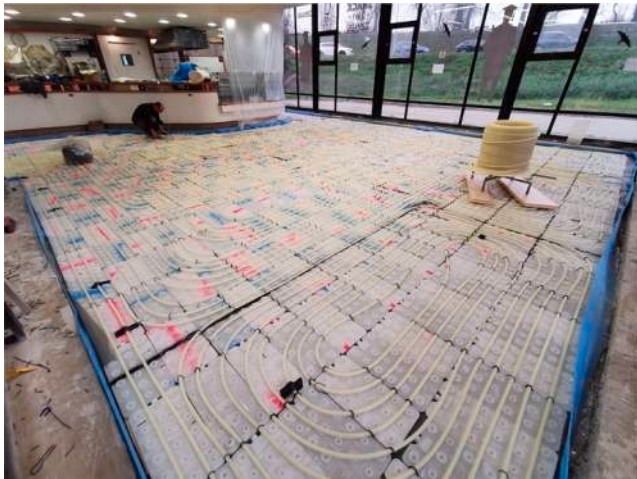
Fig. 5. Installation of the piping over PCMs.
