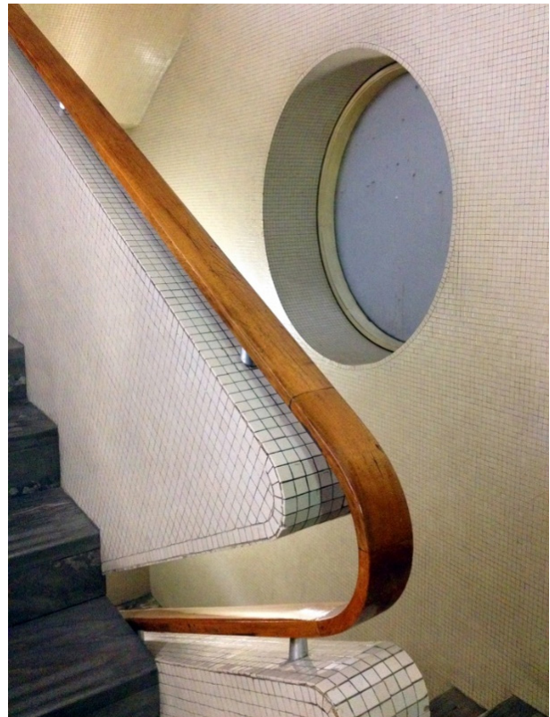
Fig. 1 Studio Ponti Fornaroli Soncini with E. Bertolaia, EIAR building, later RAI building (1939), unglazed porcelain tiles in combination with stone and wood (2021).
