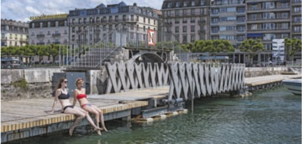
Fig.04 The flat configuration of the footbridge becomes a seamless part of the walkway. DMK Architecture Photography
