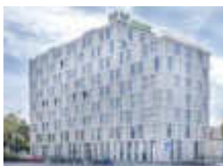
Garcia Garcia, Student Housing - Milestone Porto Asprela, Porto, Portogallo, 2019 ©Garcia Garcia *LEED Gold - "Hospitality"
