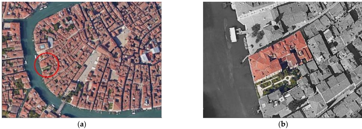
Figure 6. Palazzo Malipiero, Venice: (a) aerial view; (b) building identification.
