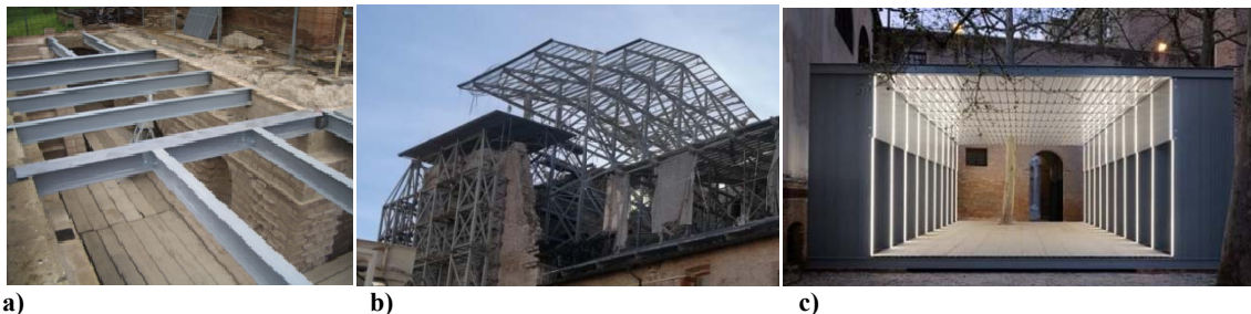
Figure 1 Examples of FRP structures, a) temporary walkway, b) post-earthquake coverage, c) Glass-House.
