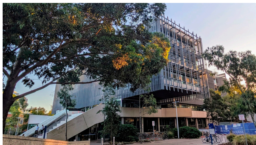
Figure 3. Melbourne School of Design (MSD) building, Melbourne, Australia.
