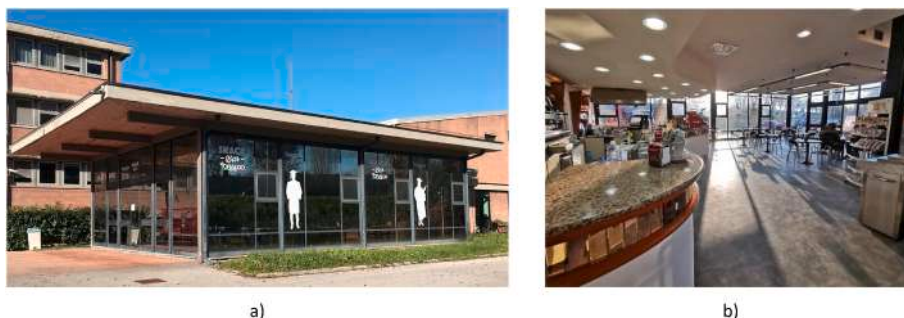
Fig. 1. View of the snack bar: a) external, b) internal.
