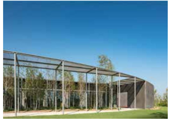
Figures 10. H-Campus new H-School Building. Credit: Marco Zanta
