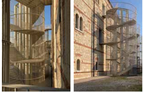
Figure 11 and 12. “Silos di Ponente” exteriors emergency exit system. 2021.
