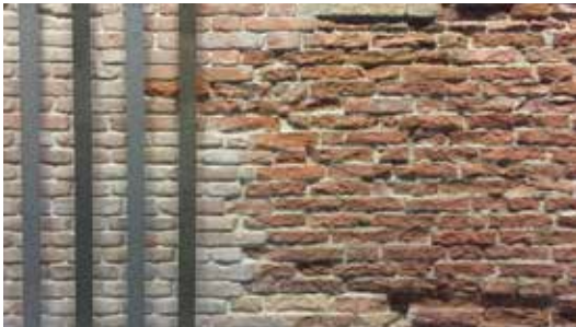
Figure 10. Interior: evidence of cuci-scuci techniques Source: Photo by the author
