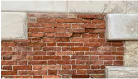
Figure 9. Exterior: evidence of cuci-scuci techniques Source: Photo by the author
