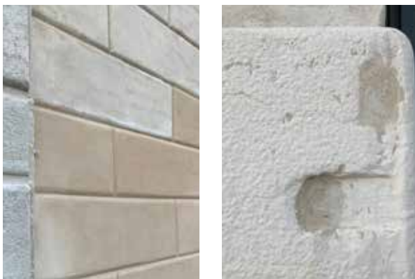
Figure 12. Exterior: surface imperfections and stuccos repaired. Source: Photo by the author
