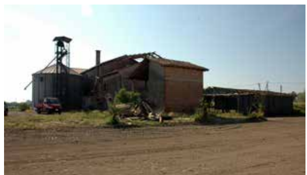
Figures 4,5 and 6. Ca' Tron estate before the intervention. Credit: ZanonAssociati Firm
