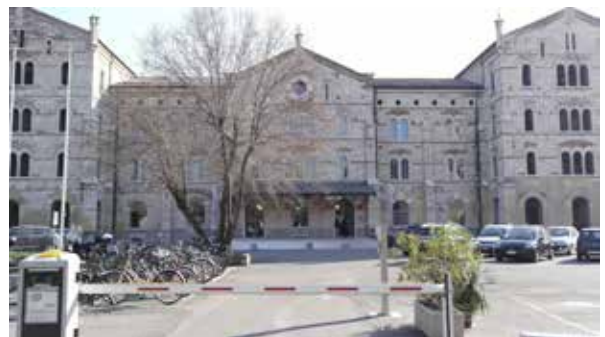
Figure 2. The former military Bakery of Santa Marta University Center. 2021
