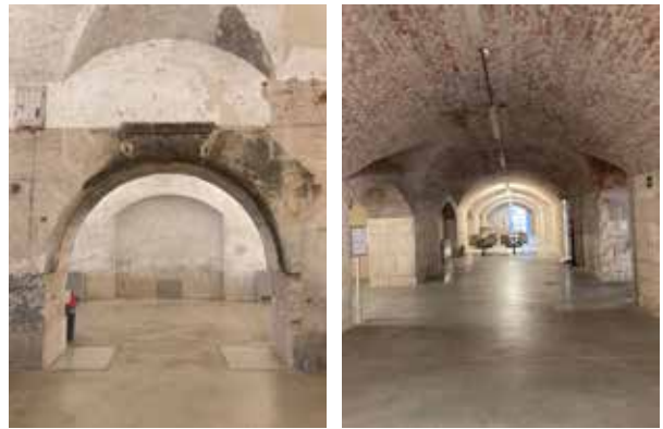
Figure 13 and 14. Former Bakery interior: ground floor. 2021.
