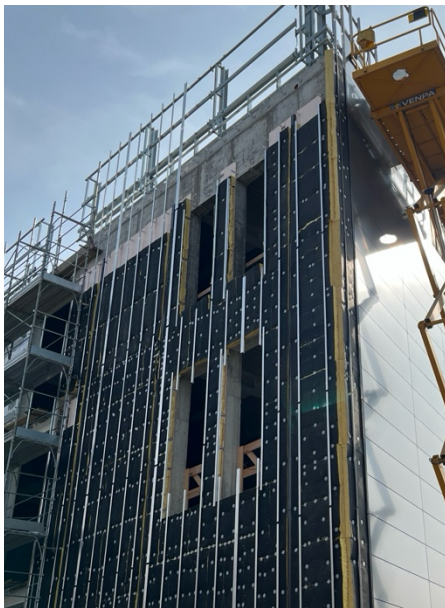
Figure 6. Example of an articulate frame substructure used for the metal cladding of the new Chamber of Commerce premises in Via Torino in Mestre.
