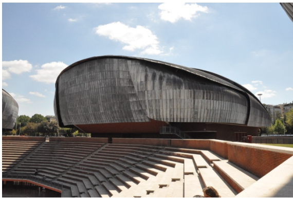
Figure 4. Lead cladding of the Music Park Auditorium in Rome by RPBW.
