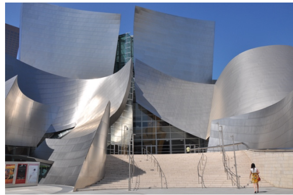
Figure 5. Stainless-steel metal-clad of the Walt Disney Concert Hall in Los Angeles by Frank Gehry.
