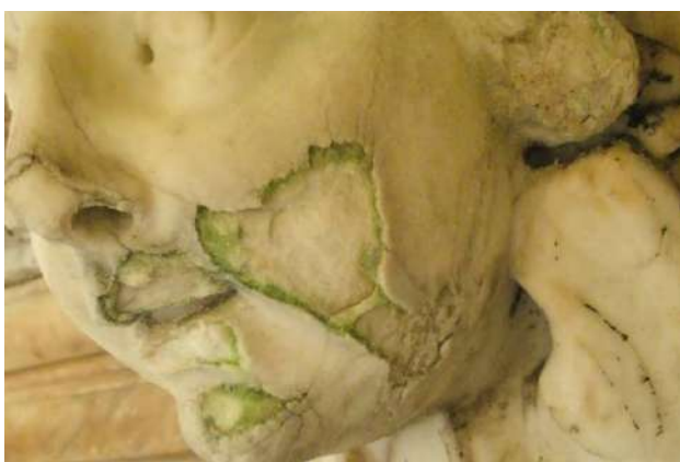
Figure 3. Detail of a cherub placed in the string course of the second order of the façade, clear example of different states of degradation of Carrara marble.
