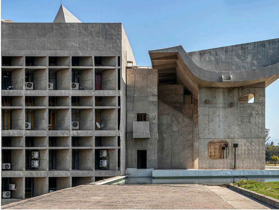
fig. 1. Palace of Assembly in Chandigarh (Le Corbusier, 1951-62), designated as a UNESCO World Heritage Site in 2016. External units of the air conditioning system on the façade. (© Roberto Conte, 2019)
