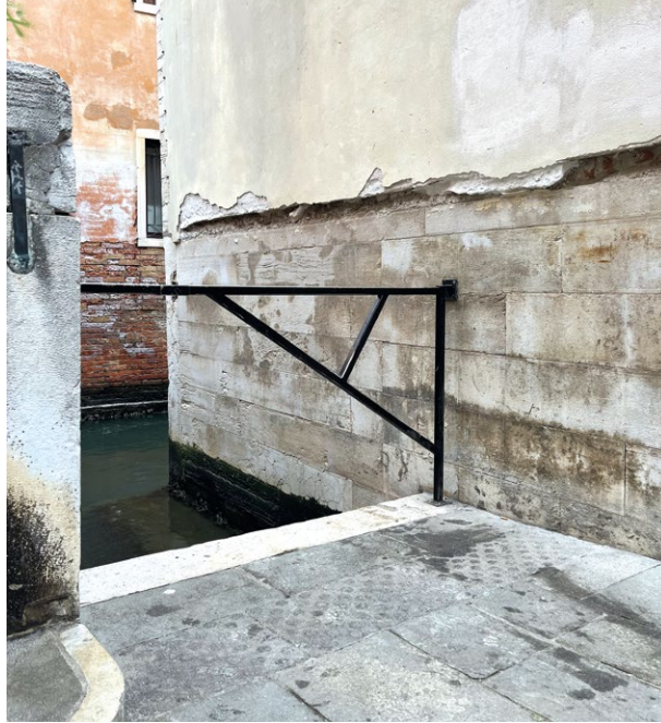
Fig.04 Extra security aid due to Tactile Indicators with no tonal contrast with the surrounding paving.
