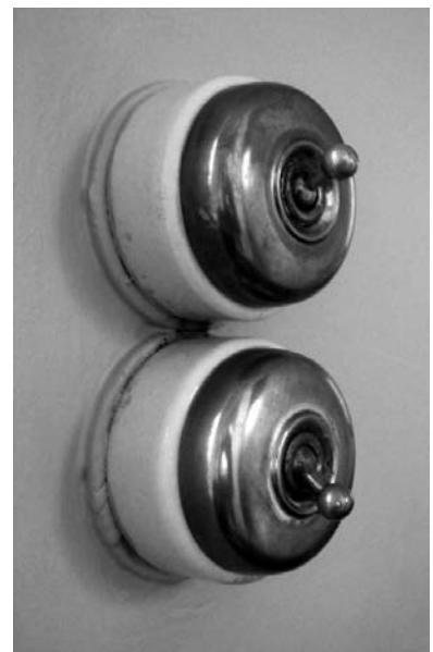
Fig. 8. Le Corbusier, La Roche house, brass switches
