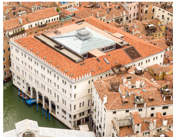
Fig. 5 The altana that replaced the rooftop proposition in the last version of the project presented in November 2012 (Source: Kasa Fue 2020, modified by the author 2025)
