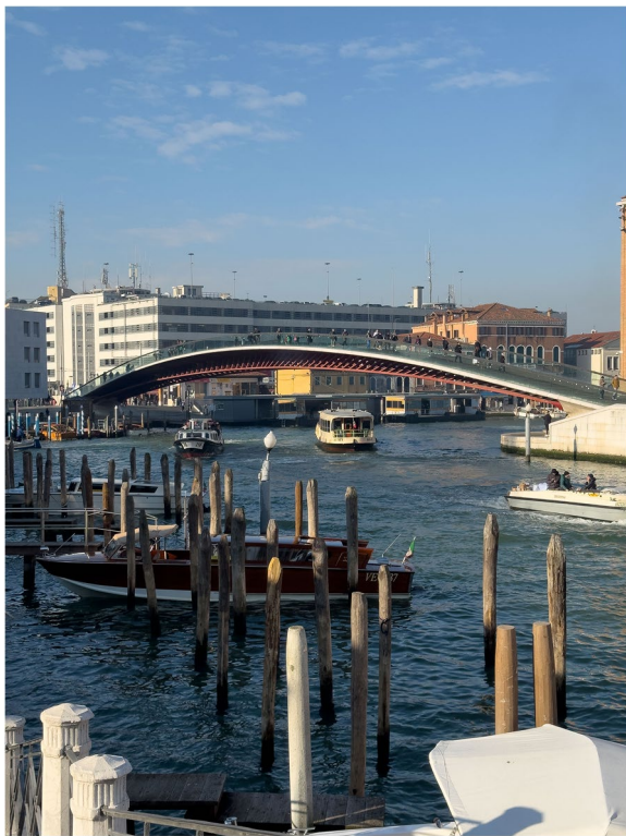
Fig. 2 Constitution Bridge (Source: the author 2024)
