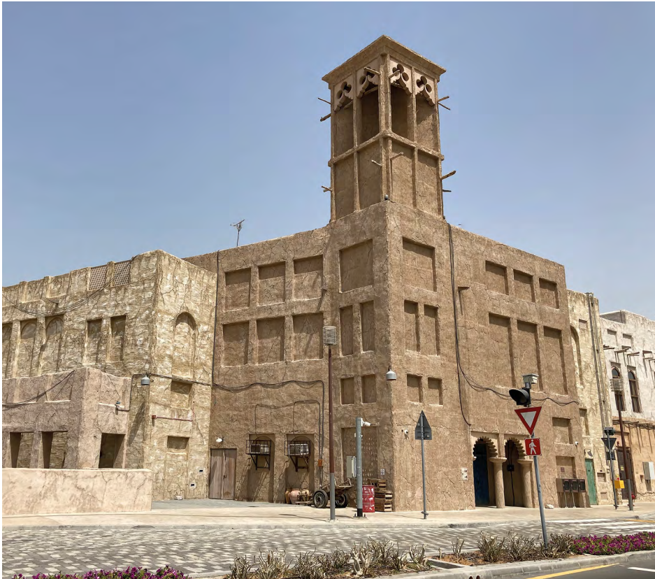
Fig. 01 A traditional Arabic building with windcatcher. C. Scanagatta
