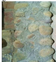
Figure 4. Photograph of an external wall section.
