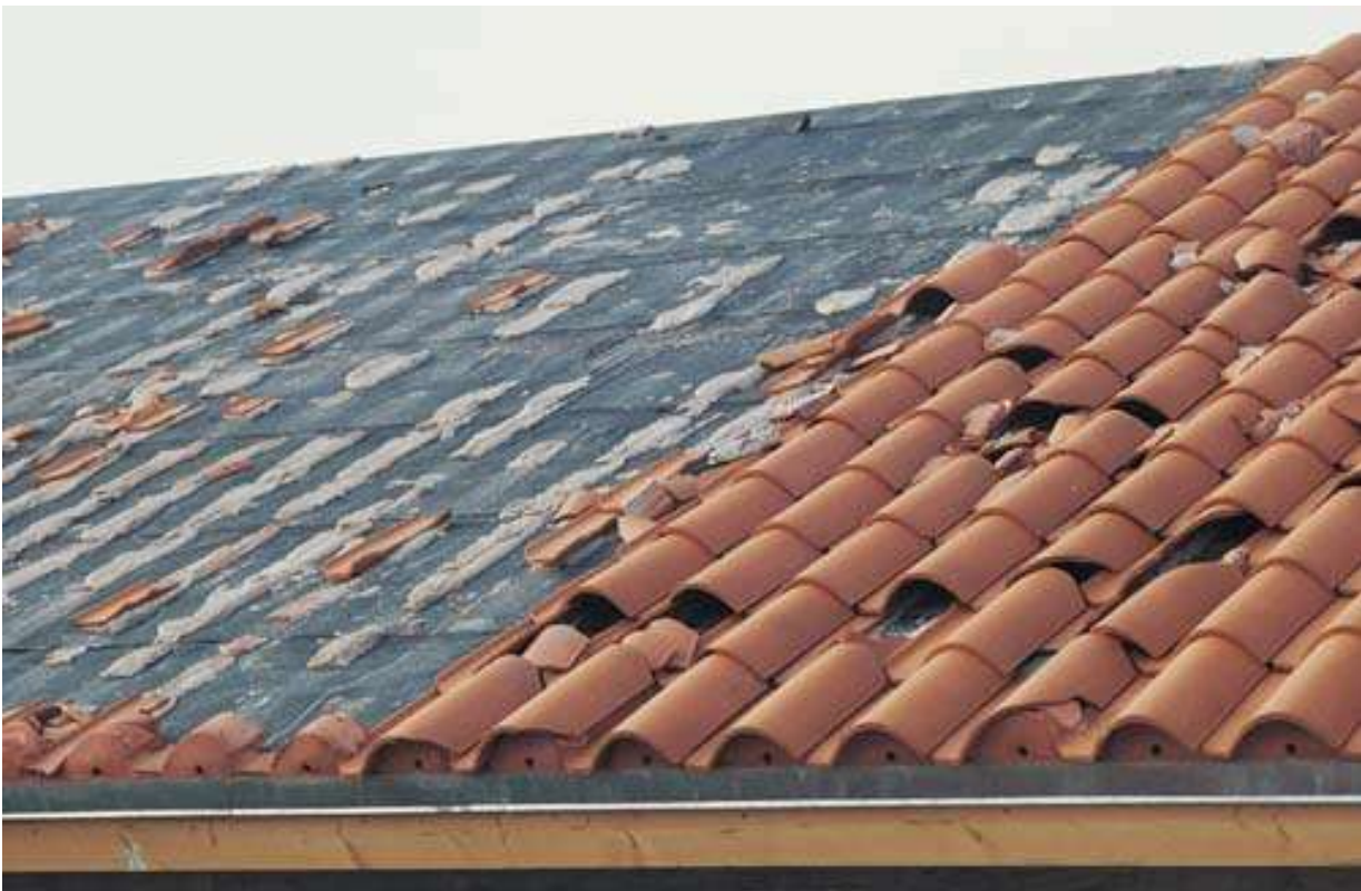
Figure 6 - After Hurricane Andrew 1992. These clay tiles were mortar-set. Three failure modes are illustrated: Separation of the mortar from the cap sheet, separation of the tile from the mortar and debris impact damage (photo courtesy of TLSmith Consulting Inc.).
