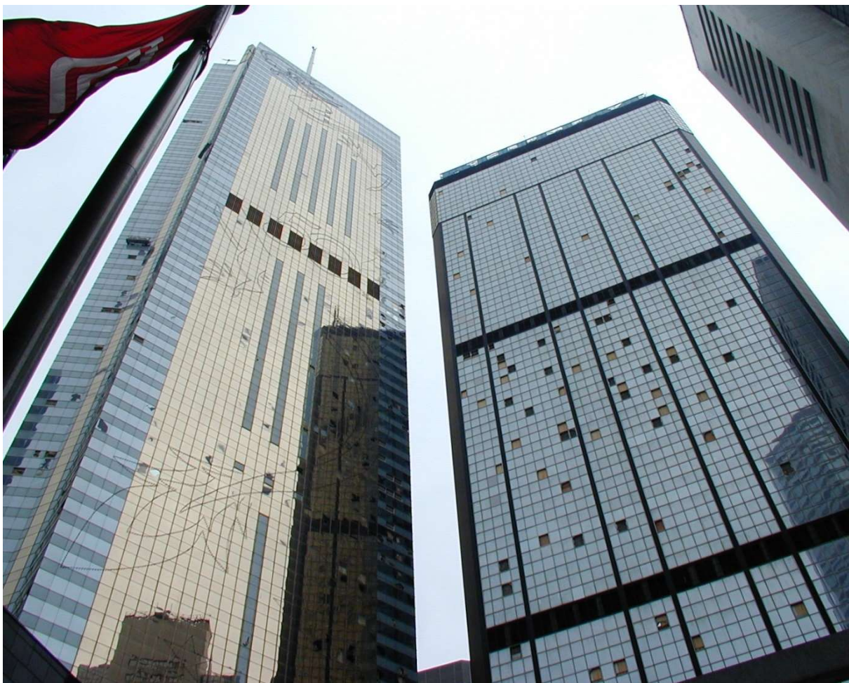
Figure 14 - Hong Kong, 1999. Typhoon York damaged the curtain walls of many buildings in Wan Chai area. Wind-borne debris caused the breakage of glazed panels in the highest tall building floors (photo courtesy of Joe Khoury).
