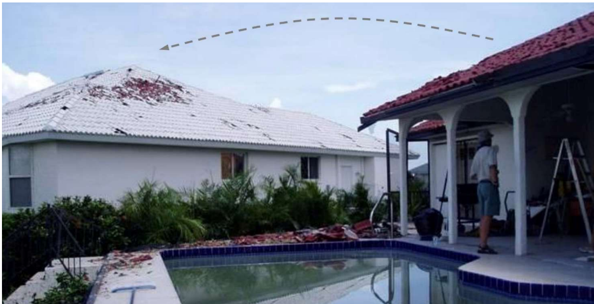
Figure 31 – Tampa, Florida. Extreme winds caused roof tile to fly and hit the neighbour house (photo courtesy of Tim Reinhold).
