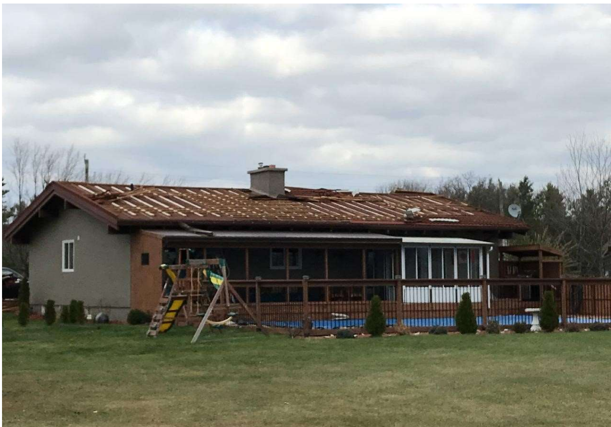
Figure 3 - Downburst winds in Dunnville, Ontario, Canada. November 11 th , 2020. Roof tile failure was recorded (Northern Tornadoes Project 2022).
