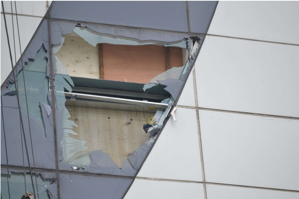
Figure 8 - Manila, 2016. When Typhoon Glenda hit the Philippines capital in 2016, building envelopes have been heavily damaged, especially the glazed panels, due to wind-borne debris impact (photo courtesy of Joe Khoury).
