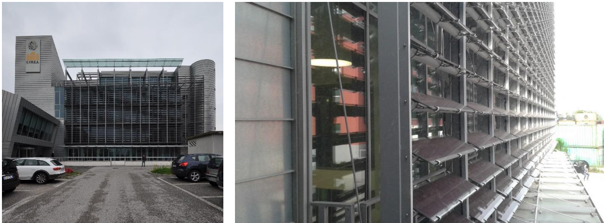
Figure 1: Example of an office building equipped with an external slat array, in this case, with a horizontal major axis and built-in PV cells, the façade is oriented approximately to the south (building headquarters of the "Citadel of Construction" in Venice, photo by the author)
