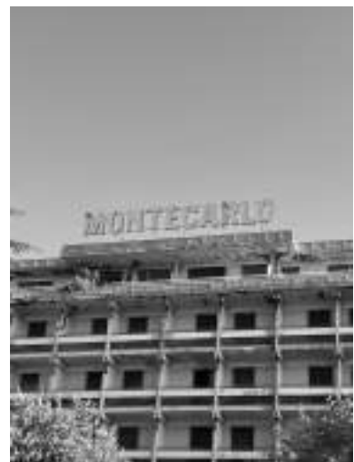
4 | The former Hotel Montecarlo, Montegrotto Terme, 2025, photo by Mauro Marzo.
