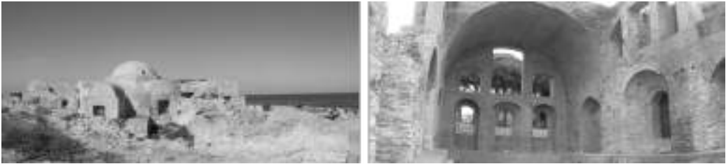
6 | View of the Roman villa of Silin near Leptis Magna and the bathing complex after restoration and roofing (Musso 2024, fig. 4).
