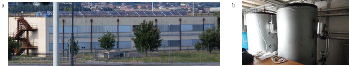
Fig. 1. (a) solar field in the roof of building; (b) hot thermal storages.
