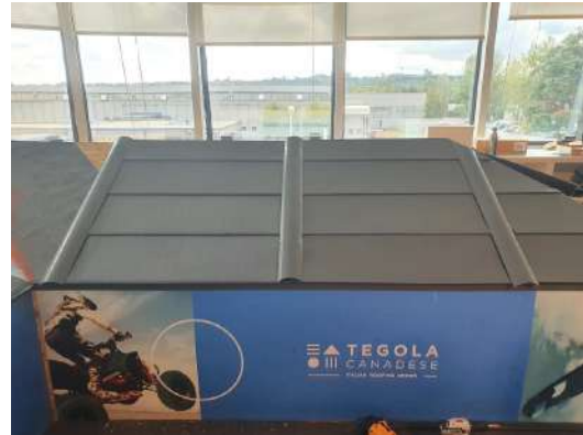
Figure 9: Installation of the BIPV system in the test room
