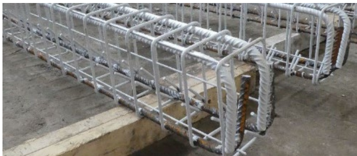
Fig. 3.3 Details of reinforcement used in the tested beams, highlighting the stirrups and compressive longitudinal rebars which were epoxy painted (From Di Carlo et al. [69])
