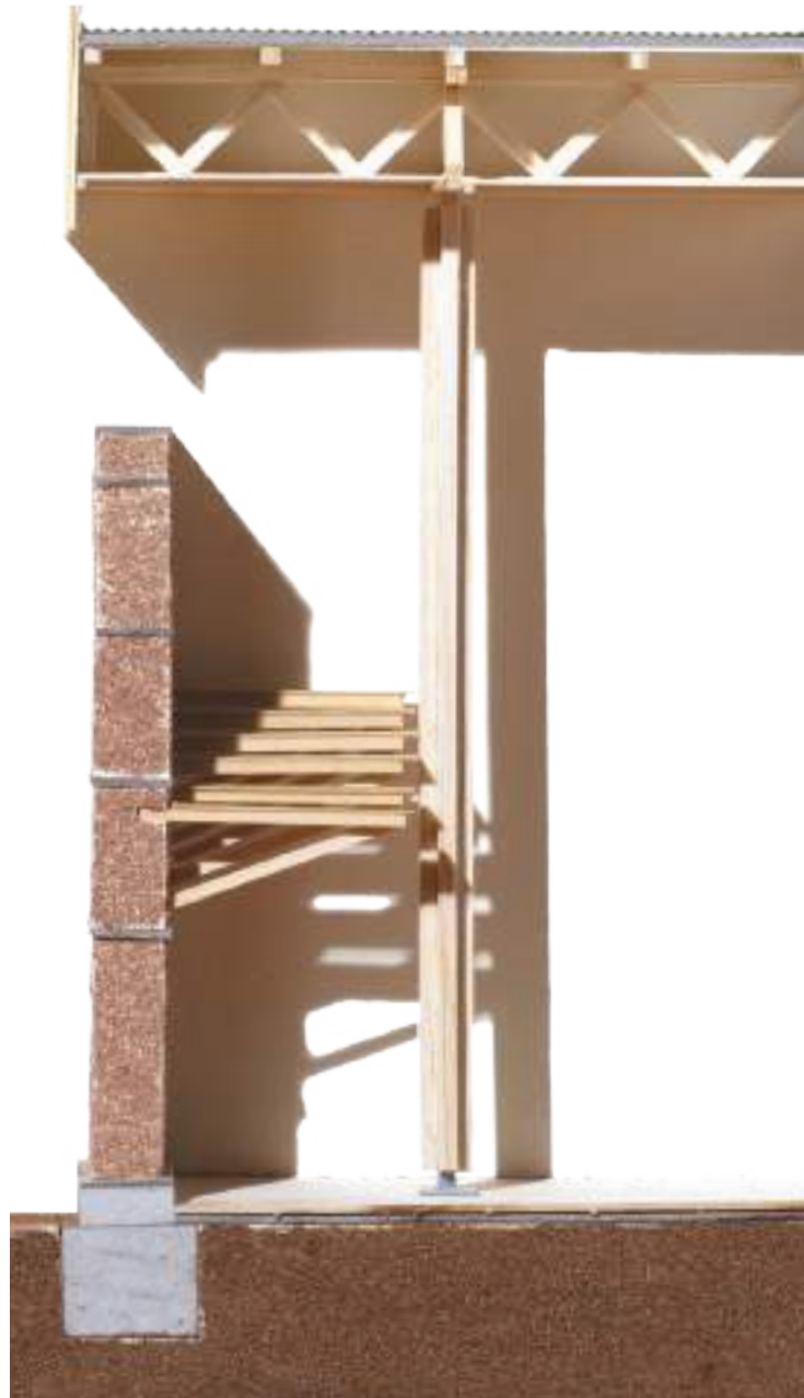
1:25 scale model in which the choice of the pisé construction technique and the large roof supported by a structure with pillars and wooden reticular beams are highlighted.
