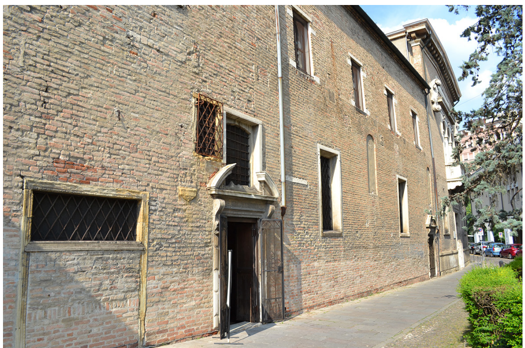
Fig. 1. Scuola del Carmine, view of the exterior: Main entrance from Piazza Petrarca.
