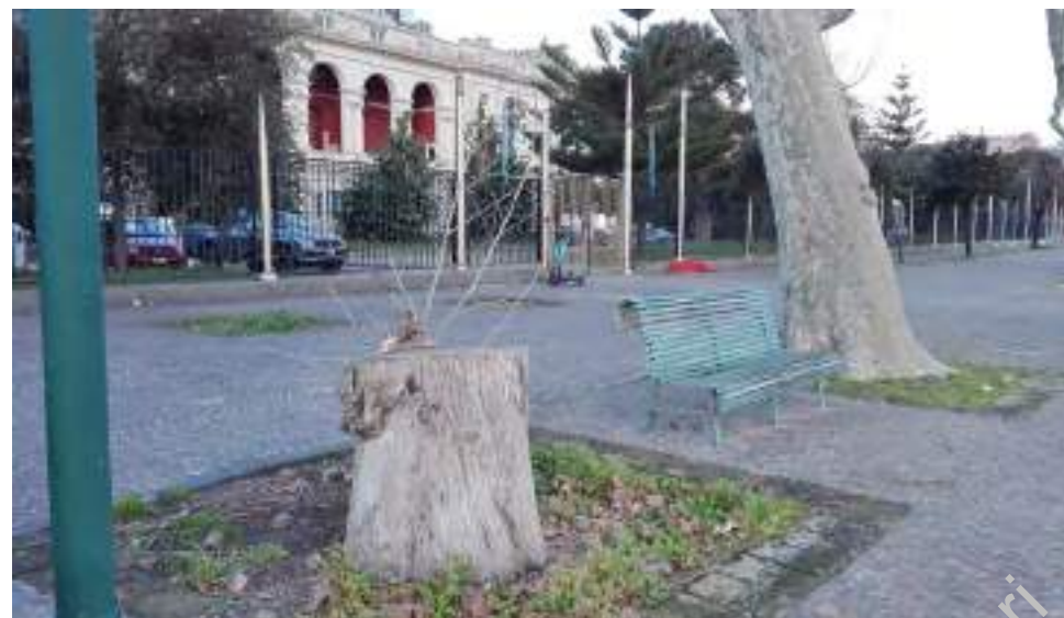
Fig. 2. Via Caracciolo, Villa Comunale side; poor maintenance of street furniture and greenery (Cuturi C., February 2023).
