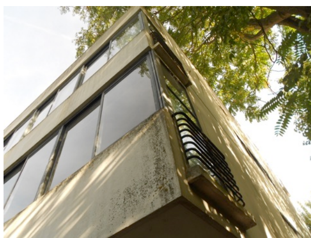
Figure 5. Detail of the South-East corner, current state [Di Resta, 2015]
