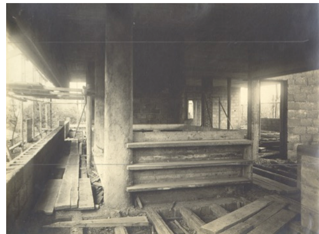
Figure 3. Internal view of the building site, first floor [FLC L1-10-3]
