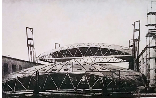
Figure 4. Experimental prefabricated bottom-up concrete shells 40x40 m span, 5 cm thickness. Developed by the LISI laboratories in Leningrad. (Davidov 1958).
