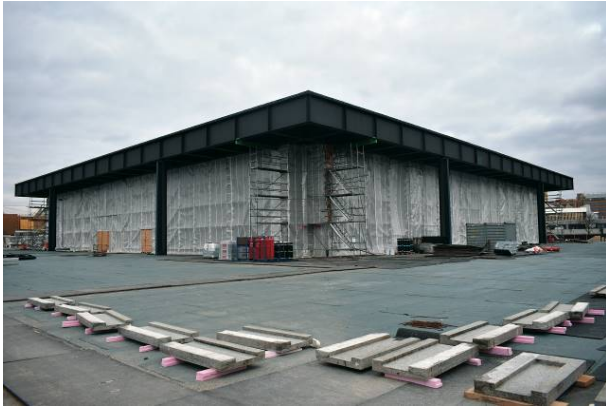
Fig. 3 Restoration site of the Neue Nationalgalerie, external view (Di Resta 2019).
