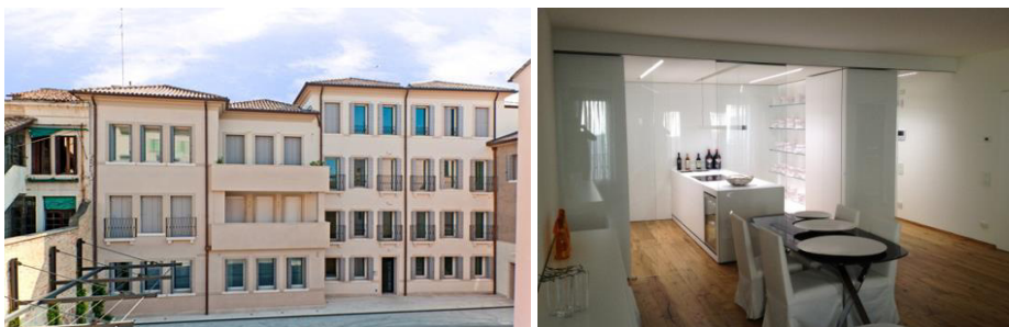
Fig. 6 The residence after intervention: a) Courtyard from west perspective; b) Typical living room in a dwelling.
