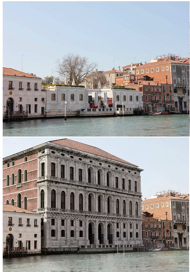
Figure 8. Comparison between the real view of the palace from the Great Channel and the hypothetic recreation of the complete façade
